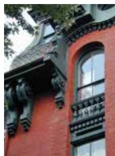
Detail, Bruce Residence
